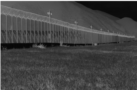
Figure 15 Example of infrared image of airport perimeter fence
