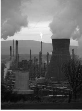
Figure 18 Example of modern petrochemical plant
